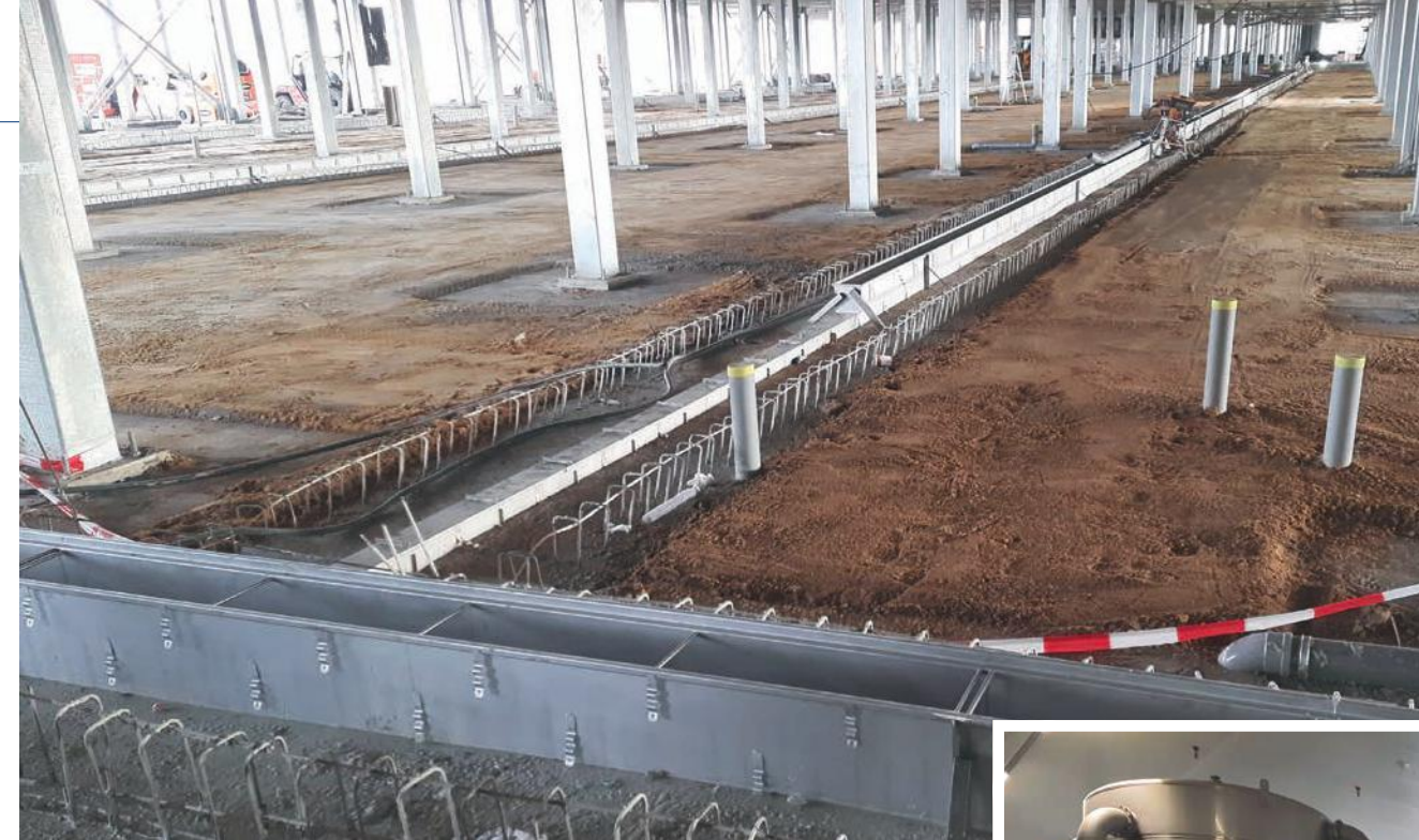
← The flume system under construction.
