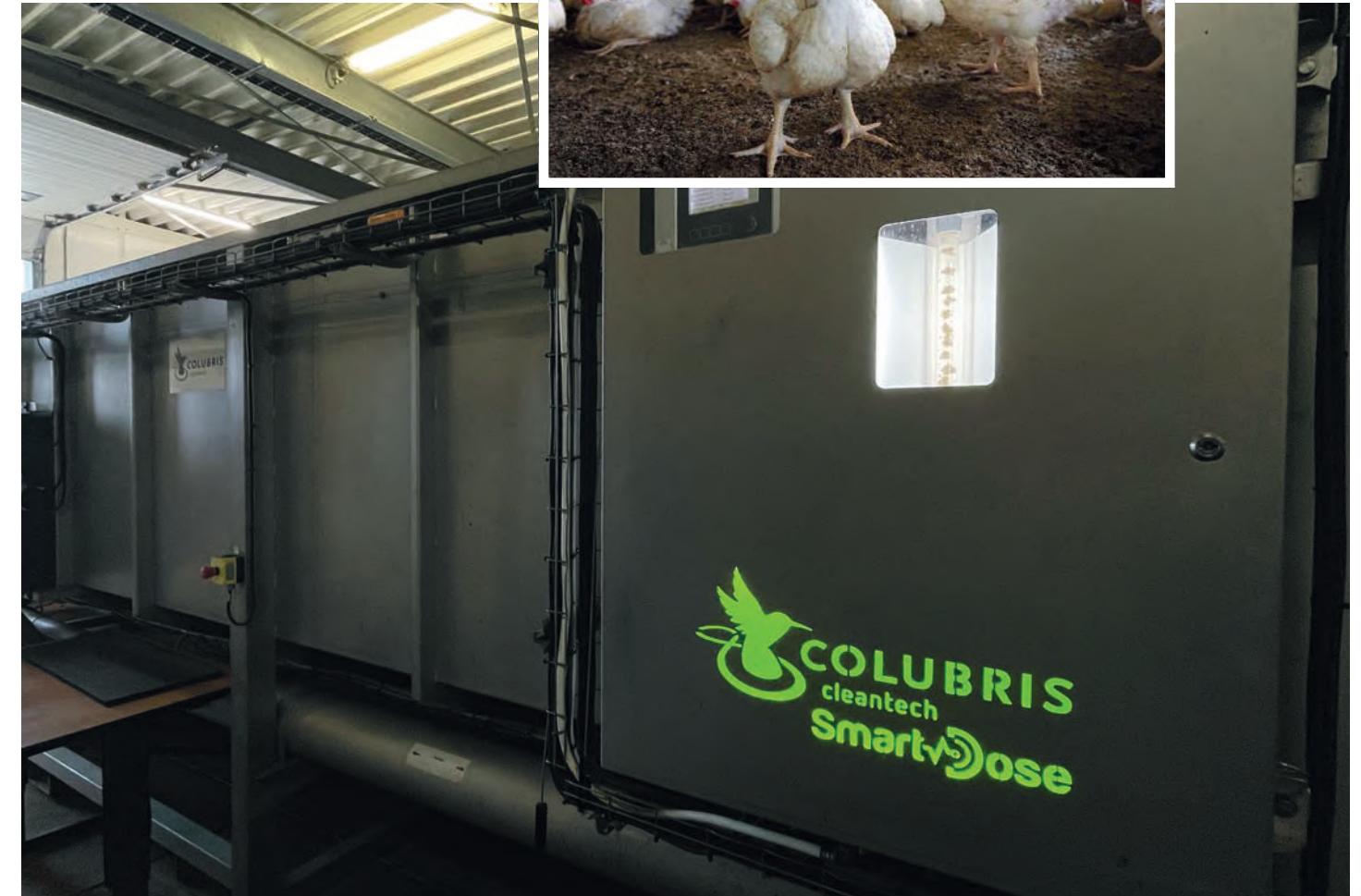
↑ At the treatment plant of Plukon in Goor (the Netherlands), SmartDose automates and optimises the dosing of coagulant in water treatment.
