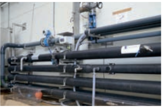
↑ The present flocculator merges small suspended solids into flocs that the flotation unit can remove from the water.
