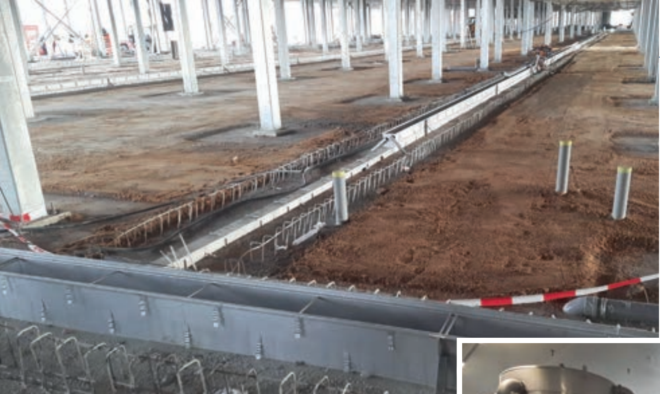
← The flume system under construction.
