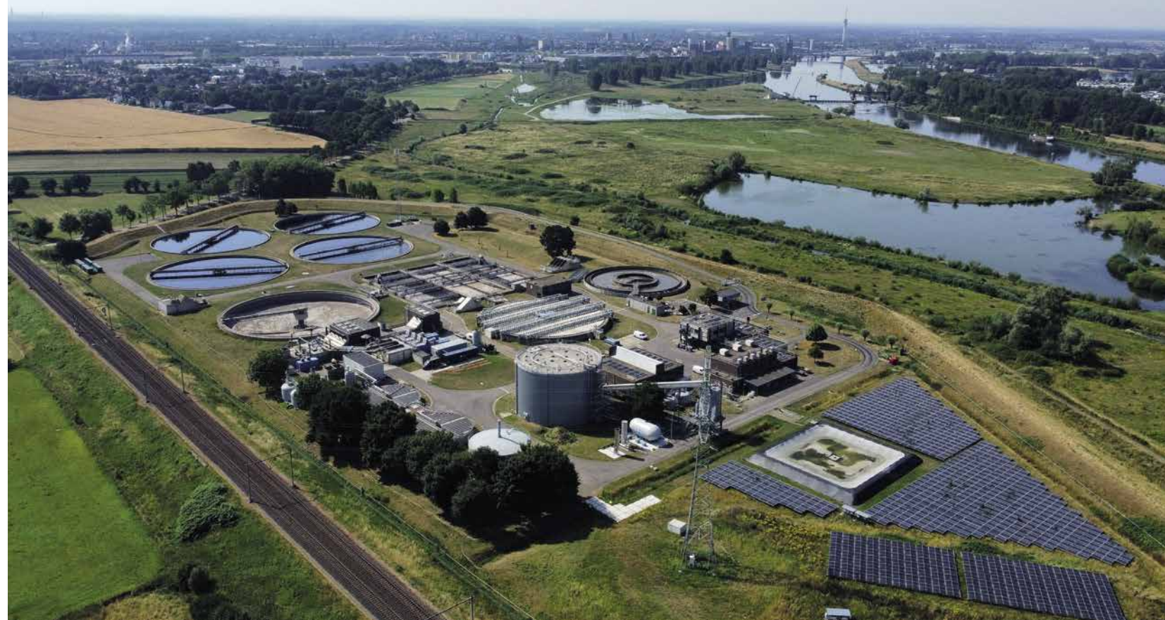
The wastewater treatment plant in Roermond, the Netherlands
